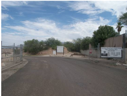
Photo 1: Site Entrance from North Prudence Road
