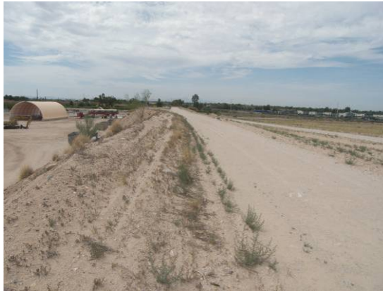
Photo 4: City of Tucson's Mullins Landfill (right)
